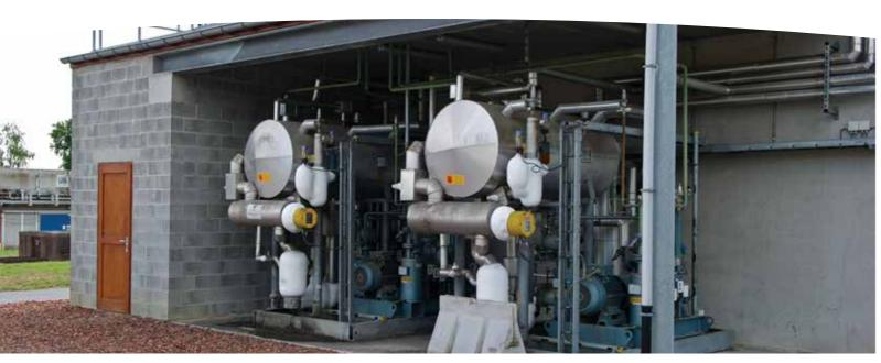
Two cooling units, alternately operating, fully independent of each other
