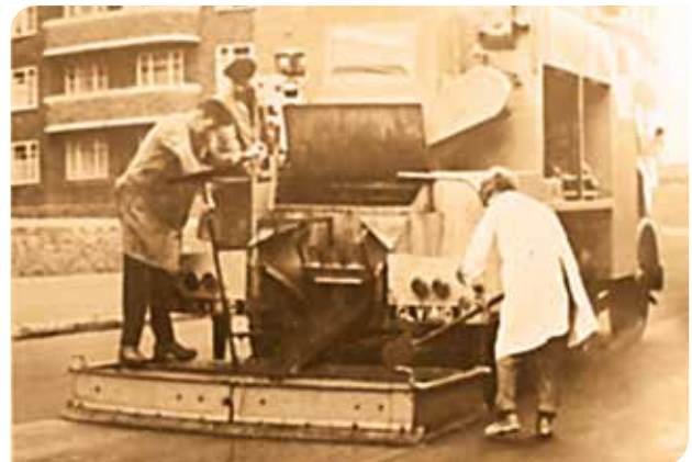
Redicote® Slurry System and Rex SlurryMatic paver circa 1965.
