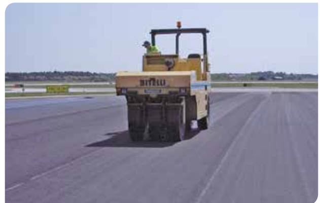
Compaction is often specified for airport jobs.
