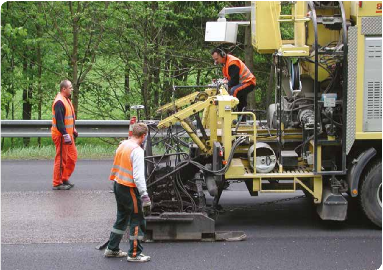
Microsurfacing in Czech Republic with Redipave phosphoric acid system.
