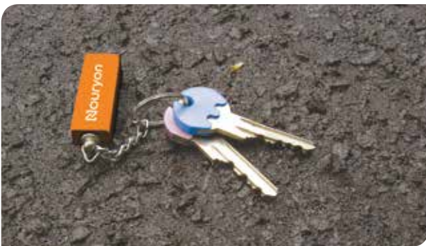
Microsurfacing provides more texture than a hot mix overlay resulting in improved wet skid resistance.
