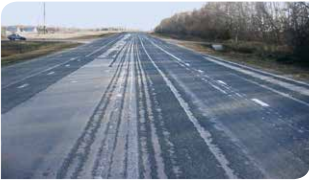
Stone losses on a surface dressing due to poor adhesion.
