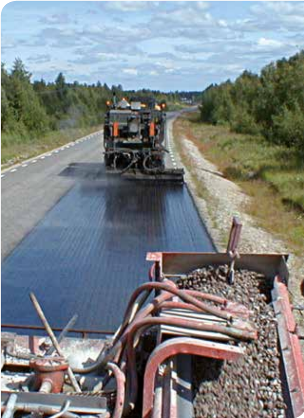
Spreading of binder and chippings during surface dressing application.
